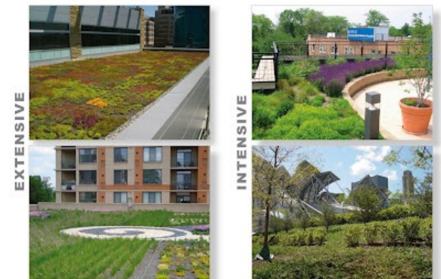
Figure 8: Aesthetic Differences between extensive and intensive green roofs (Reproduced from Ramcon Roofing, 2011)
