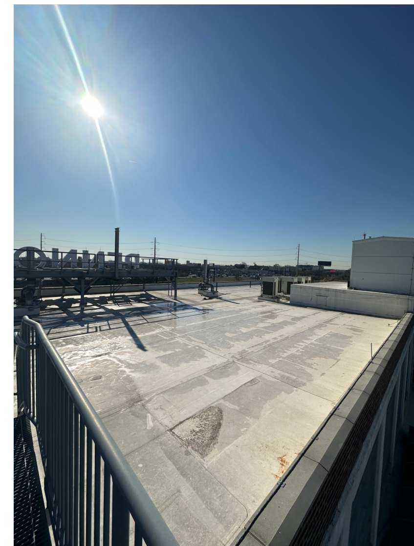
Figure 4: View of upper roof
